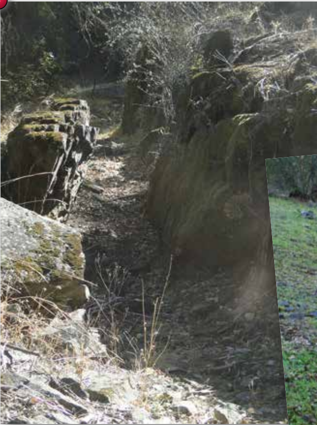
This is where the miners dug the ditch through a rock outcropping. The water flowed toward you.
